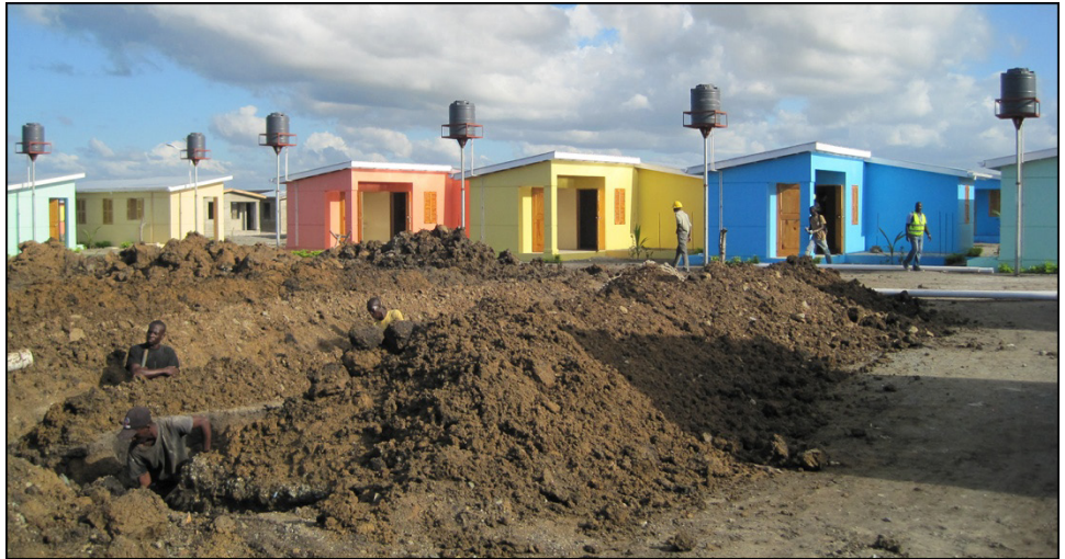
Figure 8: Unoccupied Permanent Houses, Water Distribution Towers, and Sewage System Trenches in Caracol-EKAM, Haiti, December 2012
